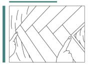
1. The subfloor must be flat and dry. In the case of panel, herringbone and mitred herringbone patterns, start fitting from the central axis of the room. For strip flooring, begin laying in a corner with the tongue against the wall.
